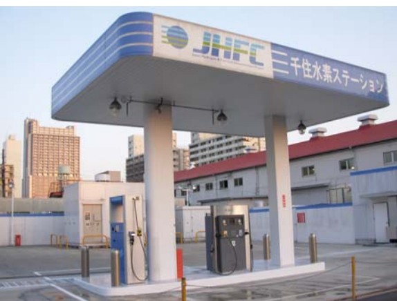
Hydrogen Station at Tokyo Gas HQ
